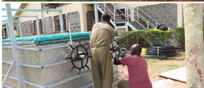
SMEP Project Migori _ Installation of Bio Gas
